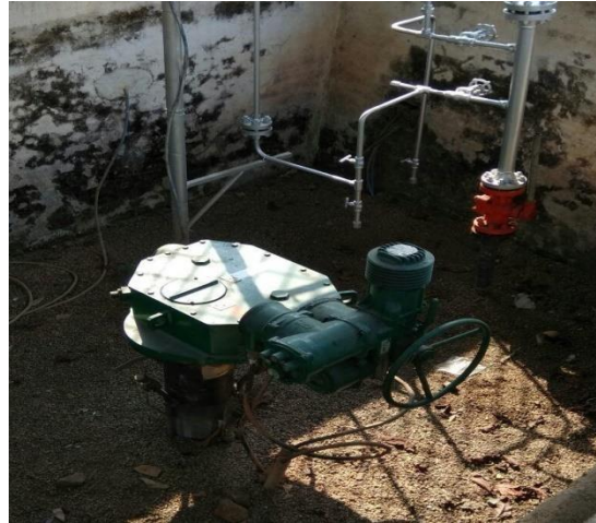
Fig 2.2 Motor operated valve
